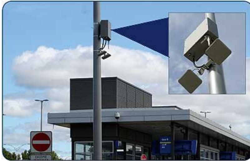
RFID interrogators mounted on lampposts at the entrance of the terminal allow the system to know when a specific bus is nearing its assigned dock (pictured behind the lamppost). Dock-mounted interrogators record the exact time each bus arrives and departs.
